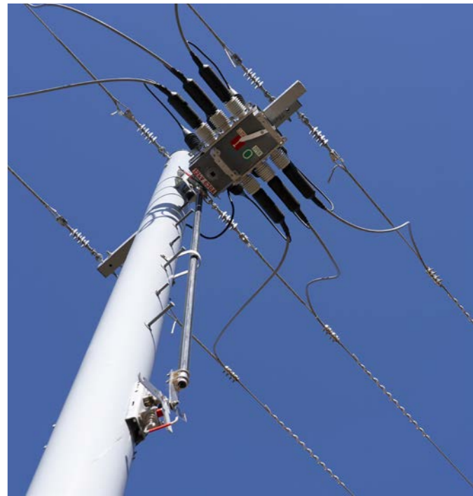
Composite pole fitted with electrical hardware and conductors, demonstrating compatibility with distribution network infrastructure and in-field performance requirements.
