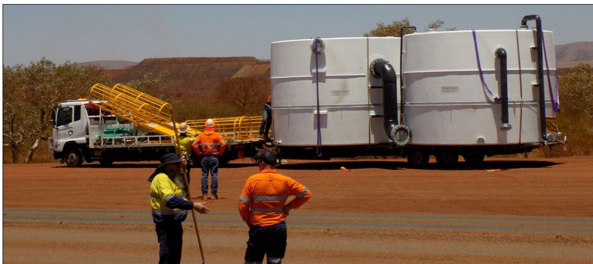
Tanks West 2 x 60,000L tanks for raw water and delivered to mine site. Image courtesy S Thompson
