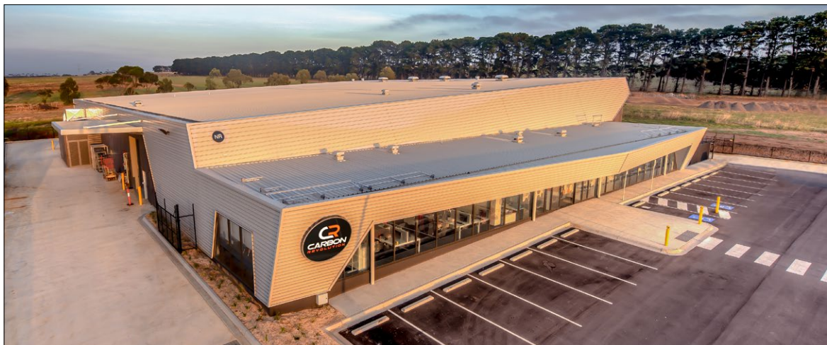
Carbon Revolution production facility (soon to be expanded) within the Geelong Future Economy Precinct in Victoria.
