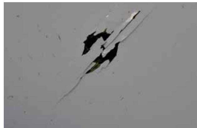
Drilling Operation Damage of Kevlar Structure (photo by Rik Heslehurst)
