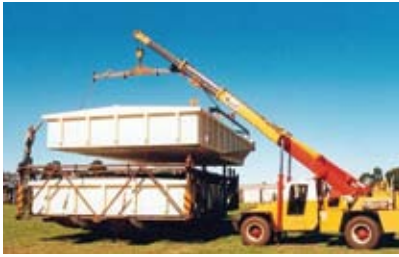
Corrosion resistant fibre composite processing tanks for CAWSE Nickel Mine
