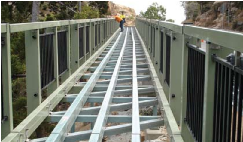
Wagners Composite Fibre boardwalks installed on Magnetic Island, Queensland
